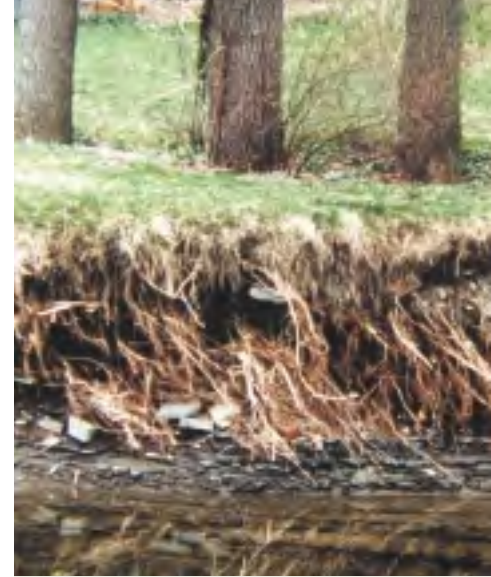
Eroding river bank
