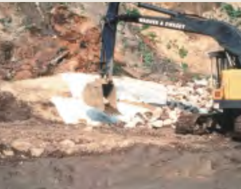
Erosion access allowance provides a route for machinery to undertake periodic repairs as well as emergency vehicles
