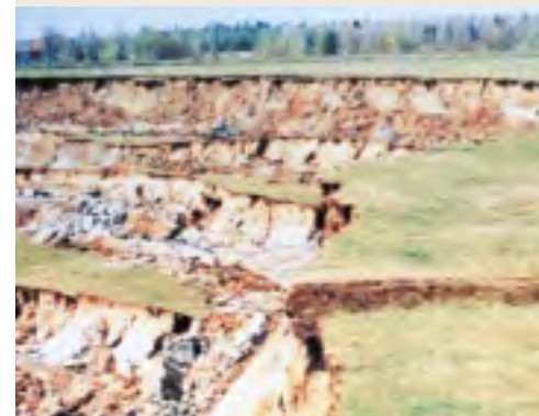
Massive slope failure
