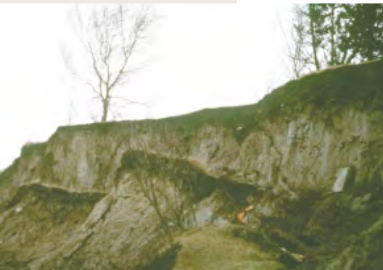
Slumping of slope on Lake Huron shoreline
