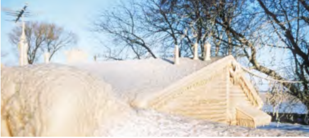
Other water related hazards – ice build up, combined with freezing wave spray on Lake Erie
