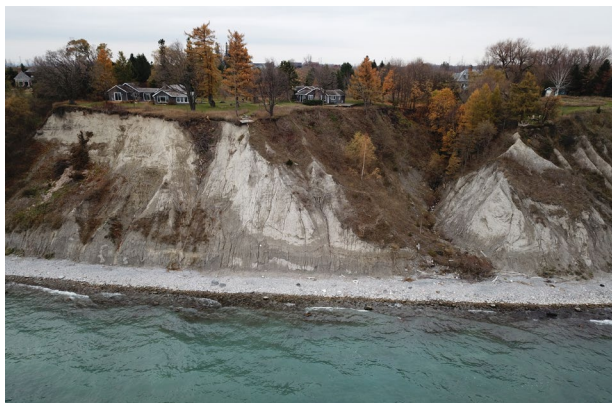
Eroding Bluffs at Bond Head
