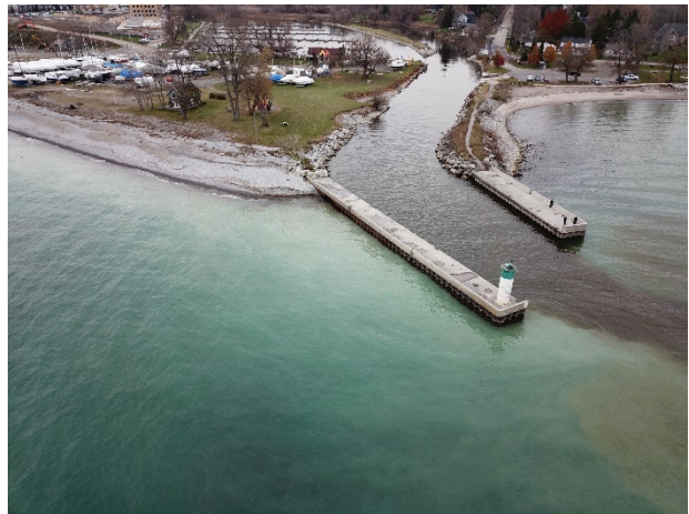
Cobble Fillet Beach and Jetties at Port of Newcastle
