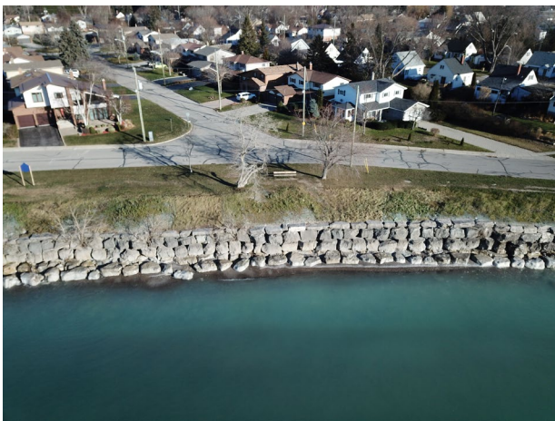
Municipal Shore Protection, Monk Street, Cobourg
